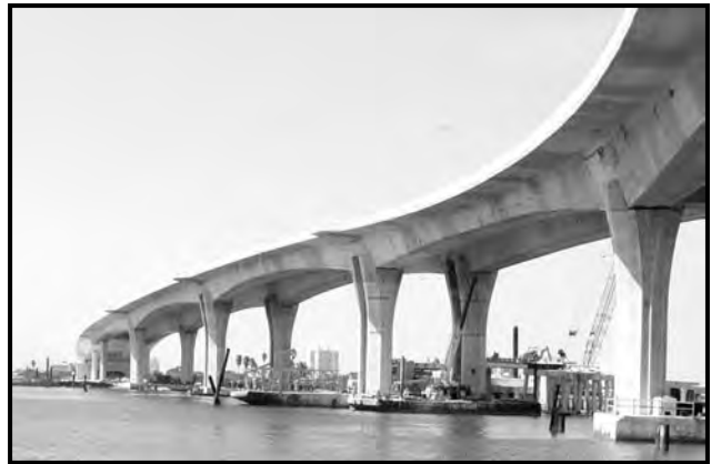
New Clearwater Memorial Causeway Bridge, 2005
